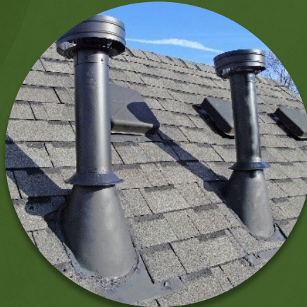
Natural ventilation: Background ventilation with stack ducts
