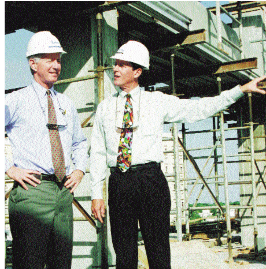
President Foote surveys construction progress of the George A. Smathers Student Wellness Center with Norman Parsons, director of Wellness and Recreation, right.
